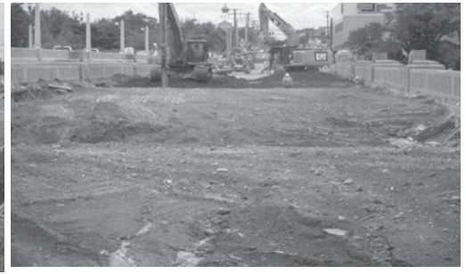
The old bridge being demolished. Where is all the dirt from???
