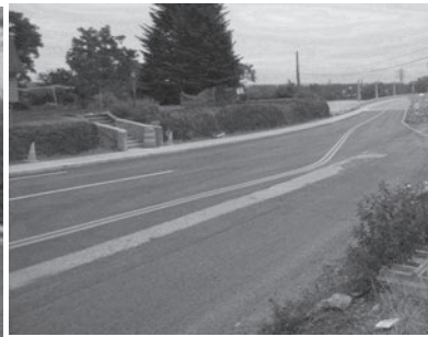
The new Waterford Bridge
