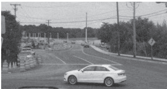
The new Waterford Bridge at New Cortland Street & 787
